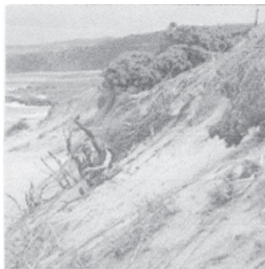
Fig. 17.7: Coastal erosion due to wave action
