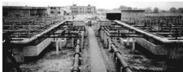
Fig. 6.11: Sewage Treatment plant under Yamuna action paln at Faridabad
