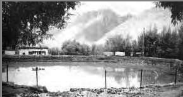
A kul leads to a circular village tank, as the above in the Kaza village, from which water is released as and when required.
