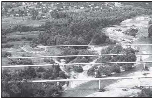
Fig. 8.17: Pipelines transporting natural gas in Ukraine
