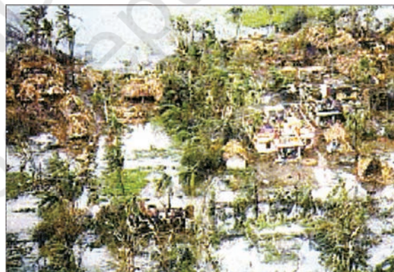
Destruction caused by a cyclone
