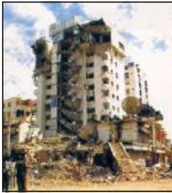
Fig. 3.3a: Destruction caused by an Earthquake in Gujarat
