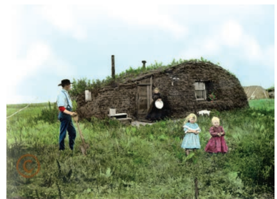
Fig.8 – Sod houses in the Frontier. (Courtesy: Fred Hultstrand History in Pictures Collection, NDIRS-NDSU, Fargo.) A typical sod house that settlers lived in when they began clearing the grasslands. Timber for houses was not available in this area.
