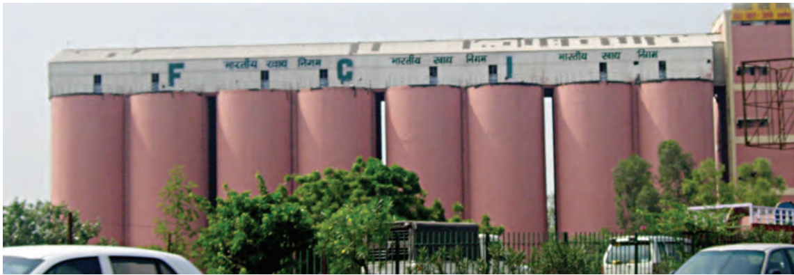
Fig. 1.10 (a) : Silos for storage of grains
