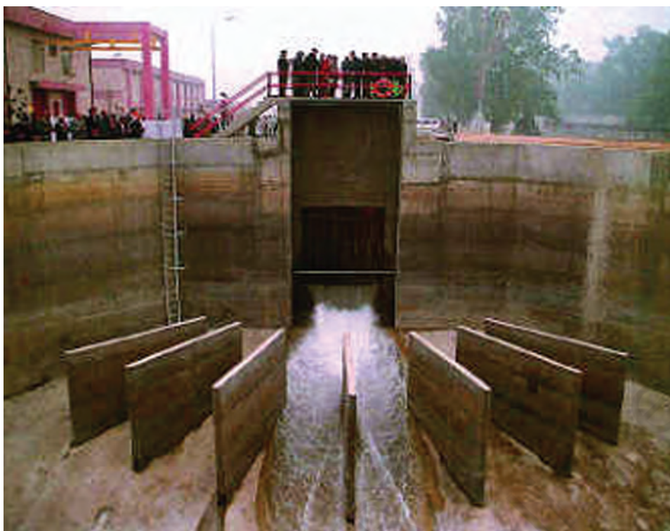
Fig. 18.10 : Water treatment plant
