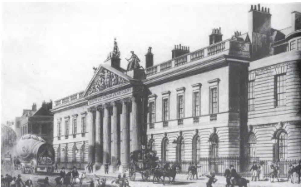
Fig. 17 – East India Company House, London.
