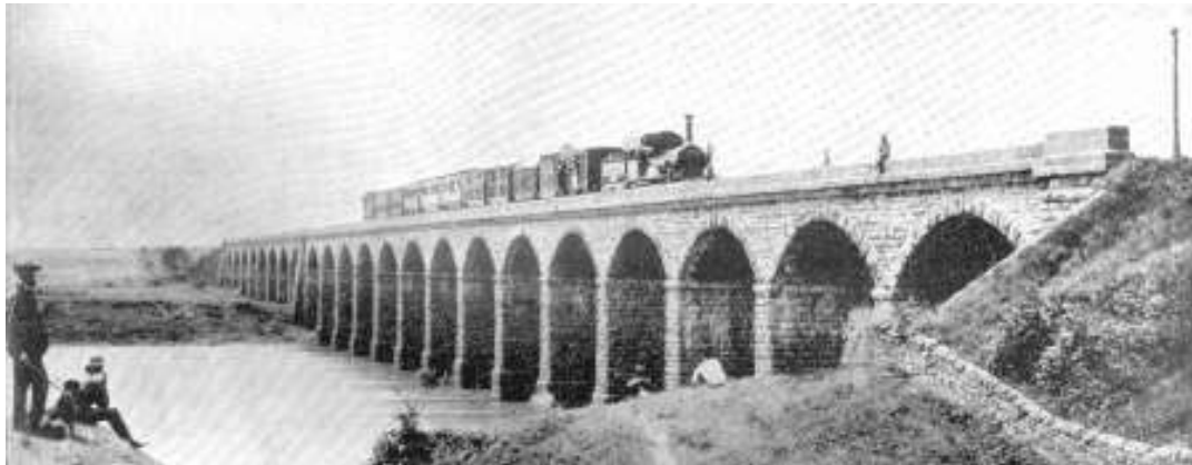
Fig. 1.4 First Railway Bridge linking Bombay with Thane, 1854
