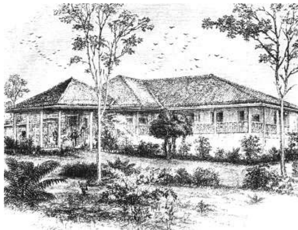
Fig. 12.23 A bungalow in Bombay, nineteenth century
